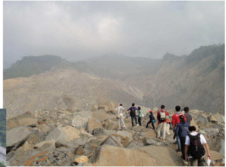
Slope failure due to rain Shiaolin Village in Kaohsiung
