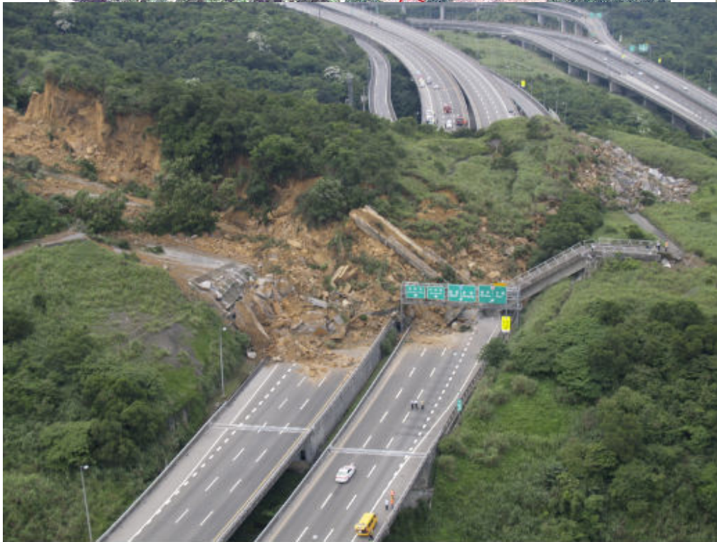
Slope failure without rain Highway No. 3 in Keelung
